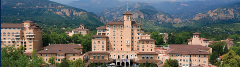
The Broadmoor Hotel Colorado Springs
